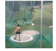
Apart from cage design, damage is often caused through misuse of the cage. Nets are often tied back to poles or hooked over rope cleats. This allows the hammer to hit the pole and the net gets squashed against the pole or torn from being tied back. The photo shows how nets are tied back to the support poles and note the left gate is open for the right handed thrower.
