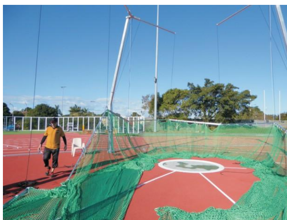
Net rails are raised by rope and tied off the cleats.
