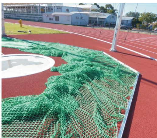
The net is evenly spaced and attached to hooks on the net rails.
