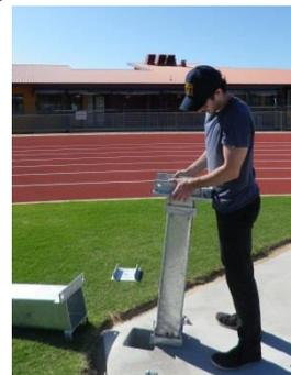
**Thor** cages do not require hire equipment to erect. The poles are assembled on the ground and raised by a winch which is supplied with the cage. There are only 3 or 4 pole holes to drill (depending on the model) and gate arches and pole bracing are not required. Thor cage footings can be installed in one day and the cage erected by two people in one day.
